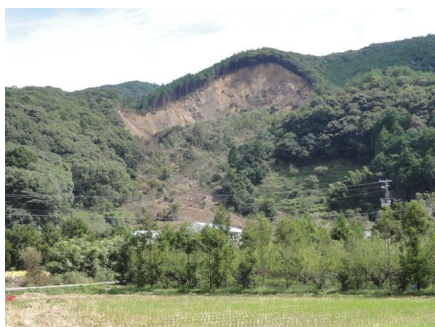
Photo 2 Large landslide at Fudono in Tanabe City
