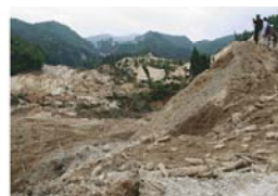
Figure 3. Field Investigations of the Aratogawa landslide caused by the 2008 Iwate Miyagi Inland Earthquake.
