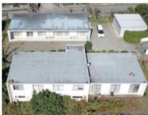
徳島地すべり観測所の施設群 Facilities of Tokushima Landslide Observatory
